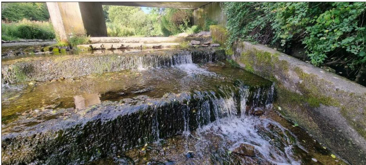
Plate 4.1 Several significant instream barriers were present in the survey area, such as the weir at site A10 on the Dinin River (passable to salmonids under higher flows but likely impassable to Lampetra sp.)
